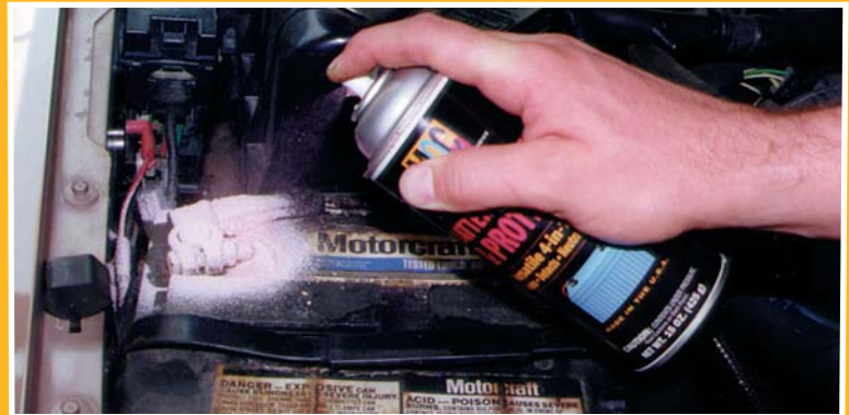
Battery-Cleaning Service in Process
